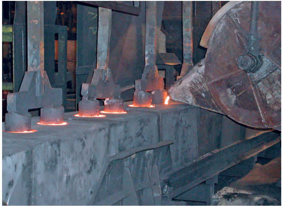
Molten cast iron is poured in the annular spacing between the steel stubs and anode stub holes
